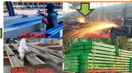
FINISHING AND PAINTING
